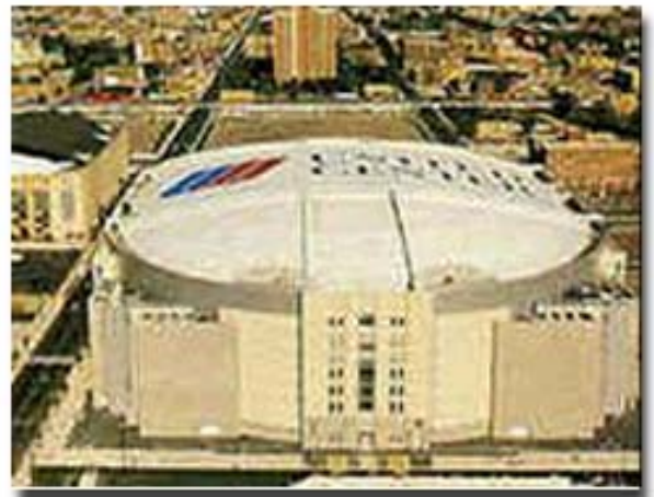
The United Center in Chicago
